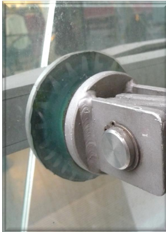
Edge Stability and Potential Cause of Blemishes in Laminated Safety Glass
